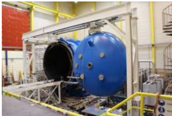
Thermo Vacuum Test Facility for VSSC (ISRO)
